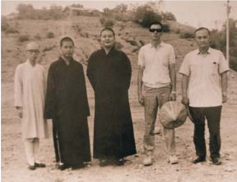
With Venerables Tzu Hui and Hsin Ping (left) at the construction site of Fo Guang Shan, after overgrowths of jute and bamboo were cleared.
